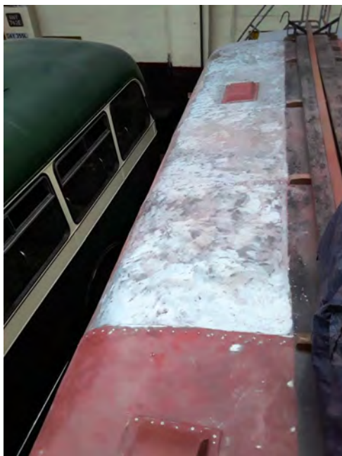
Lower left: The offside roof of 243 prepared for painting.
