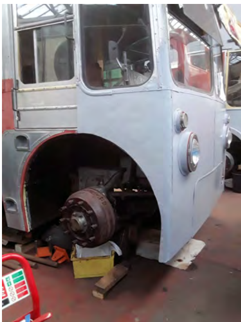
Upper right: 243's front wheel arch panel refitted and etch primed.
